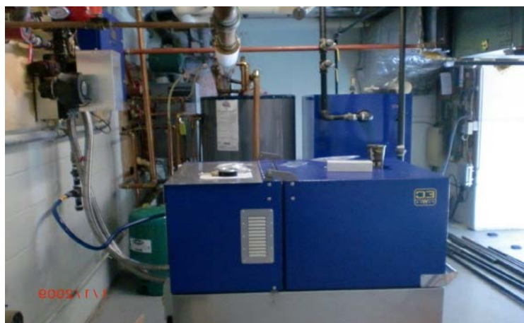
CHPP Unit, Bell St, Smiths Falls
