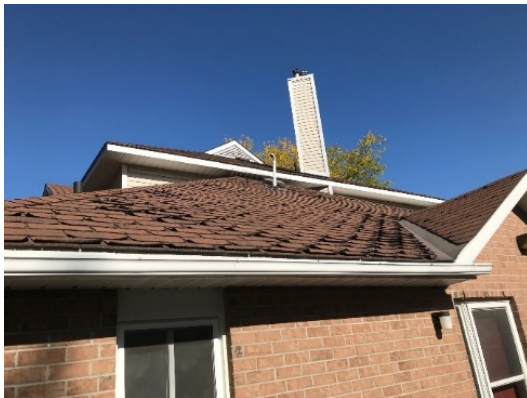
Empress Avenue Roof – Before
