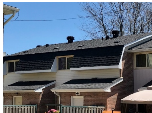
Empress Avenue Roof – After
